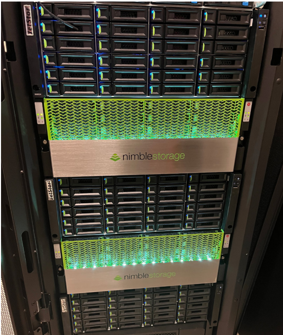
Three JetStor 824iXD Arrays at the Vilas County data center
